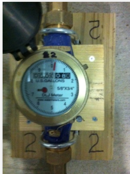
Figure 8. Two water meters purchased and installed on March 20 th , 2014 to measure pen wash down water additions to manure volume. Initial meters readings were 126.6 and 80.2 gallons for meter 1 and 2.
